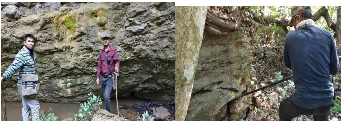
Photo: Various surface exposure of Sylhet limestone along Sukura Nala as well as nearby Kopiliconnecting road. Surfaces are weathered due continuous water and biological activity
